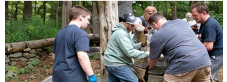
Cemetery Restoration GCBW6G4 Rhode Island
